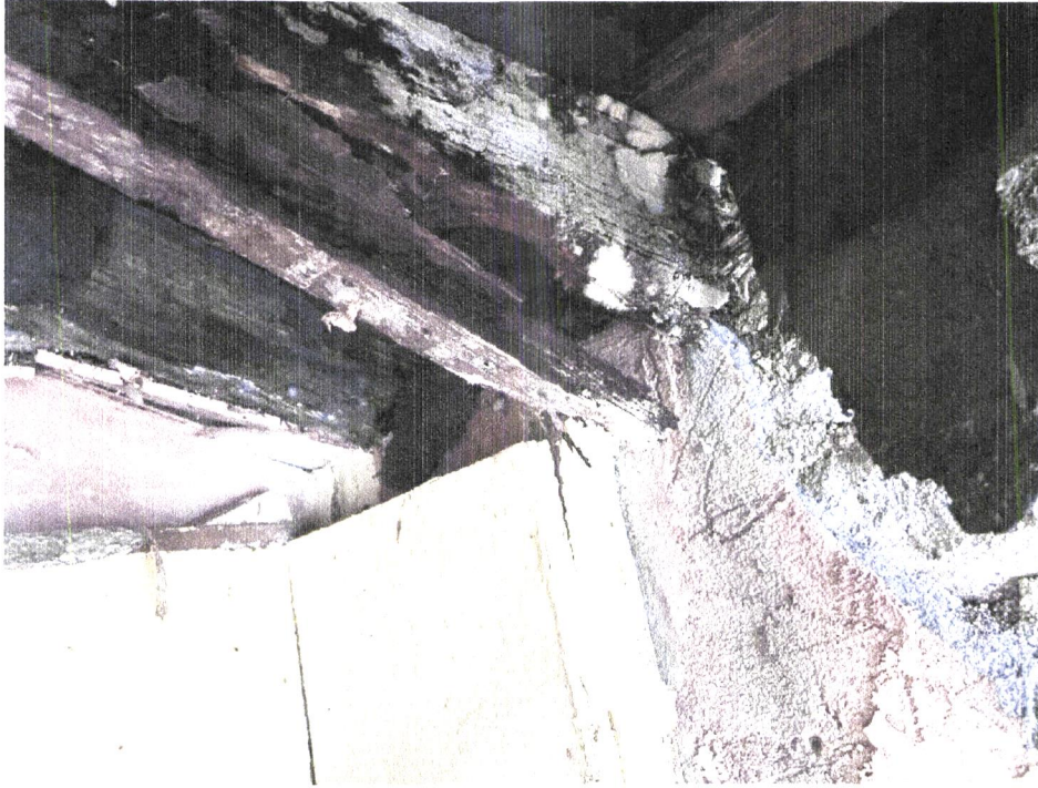
Photo 9: Rotting/loss of end bearing to timber rafter
