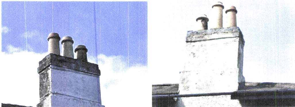
Photo 4: Close view of cracked smooth render and damaged/cracked chimney pots to chimneys
