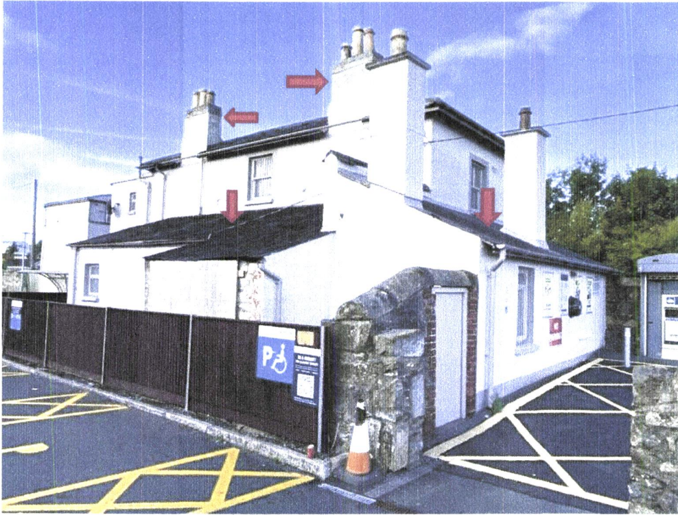
Photo 1: General view of monopitched (lean-to) roofs and chimneys attached to the Administration building
