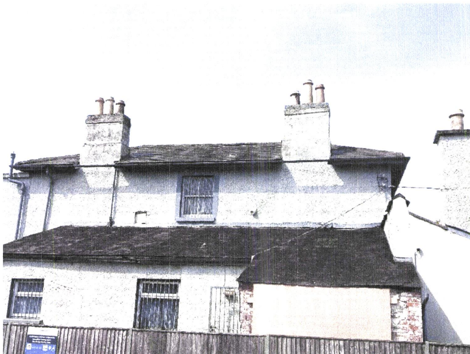
Photo 2: General View of East facing roofs and chimneys. Note bitumen coating to slates on monopitched roof
