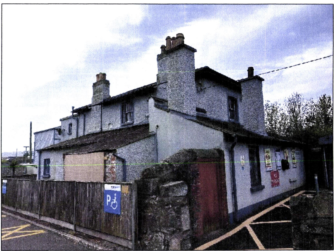
PHOTO OF MONOPITCHED ROOFS TO BE REROOFED
