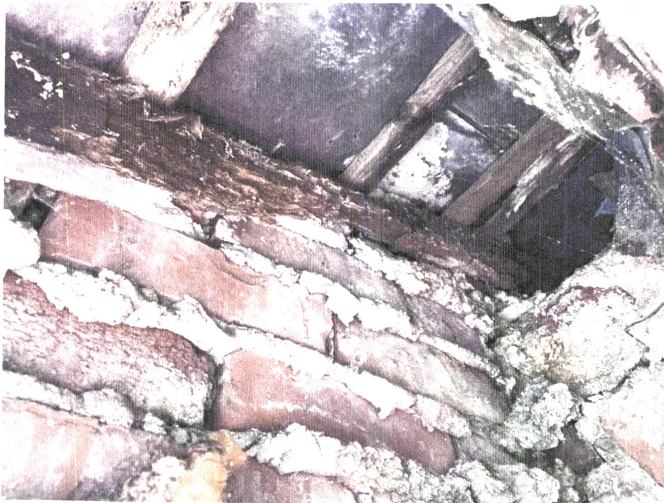
Photo 8: Rotting/decayed timber rafter
