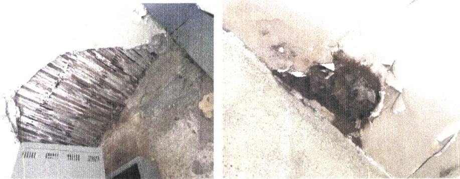
Photo 10: Missing sections of plaster to ceiling due to water ingress
