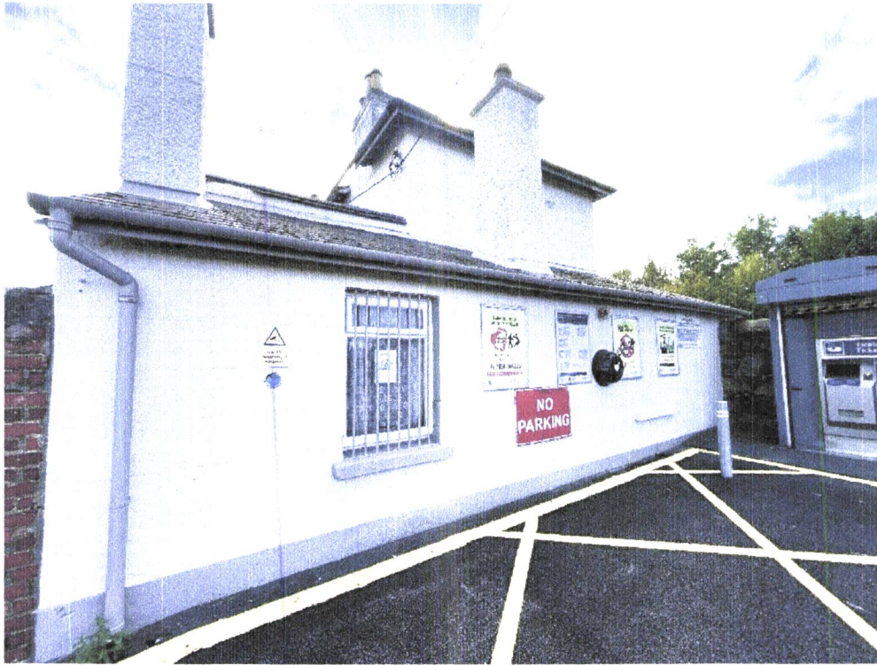
Photo 3: General view of North facing roof
